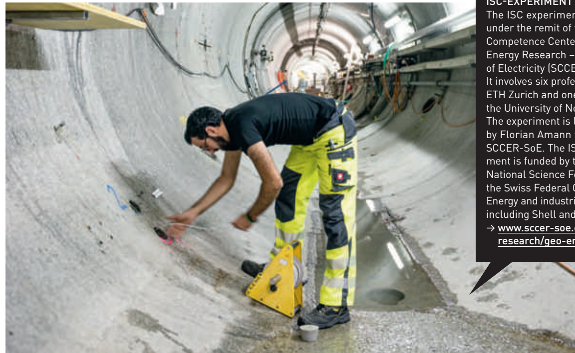
Team member Reza Jalali carefully feeds a fibre-optic cable into a borehole.
